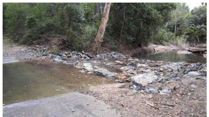
Watercourse crossings, like this one at Stony Creek Byfield, are designed to facilitate fish movement
